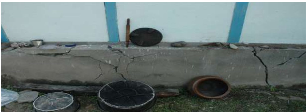
(Houses with damaged foundations – only the wooden structure on top are intact, even though dislocated from the foundation)
